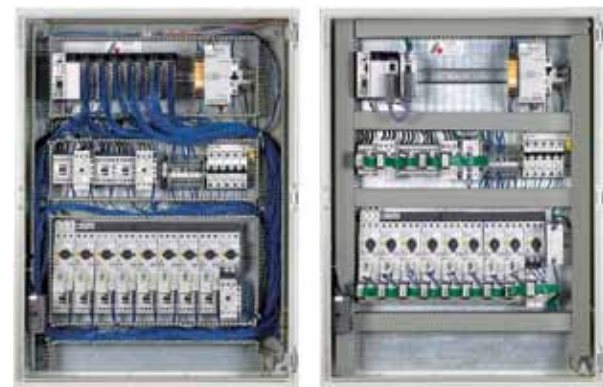
Figura 1. Panel de control tradicional, panel de control SmartWire
